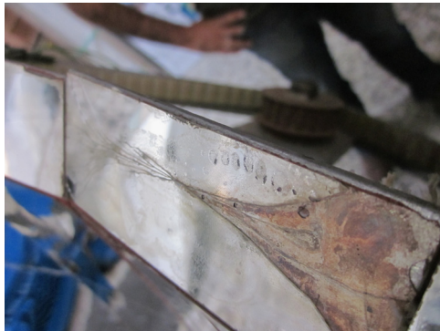
Fig. 22. Glass-cover breakage with glass-cover losses and silver corrosion, after natural aging.
