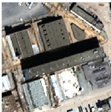
Fig. 16. The image subset used for the calculations has a large shadow cast by the building in the middle of the image.
