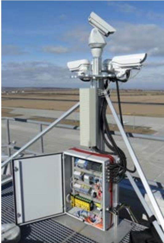
Figure 11: Panorama camera and PTZ setup on top of the Erfurt Control Tower
