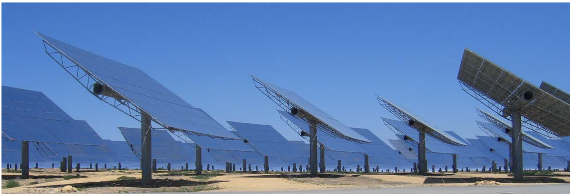
Figure 3: Heliostats with mirror planes of 120m 2
