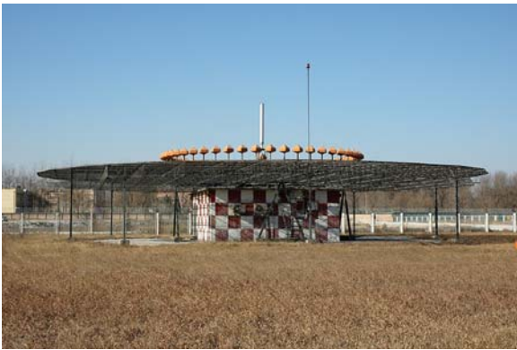
Figure 3 Typical DME station combined with a VOR (Photo by Yaoleilei).
