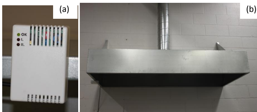
Figure 68 Safety measures: (a) Hydrogen leak sensor (b) Air extractor.
