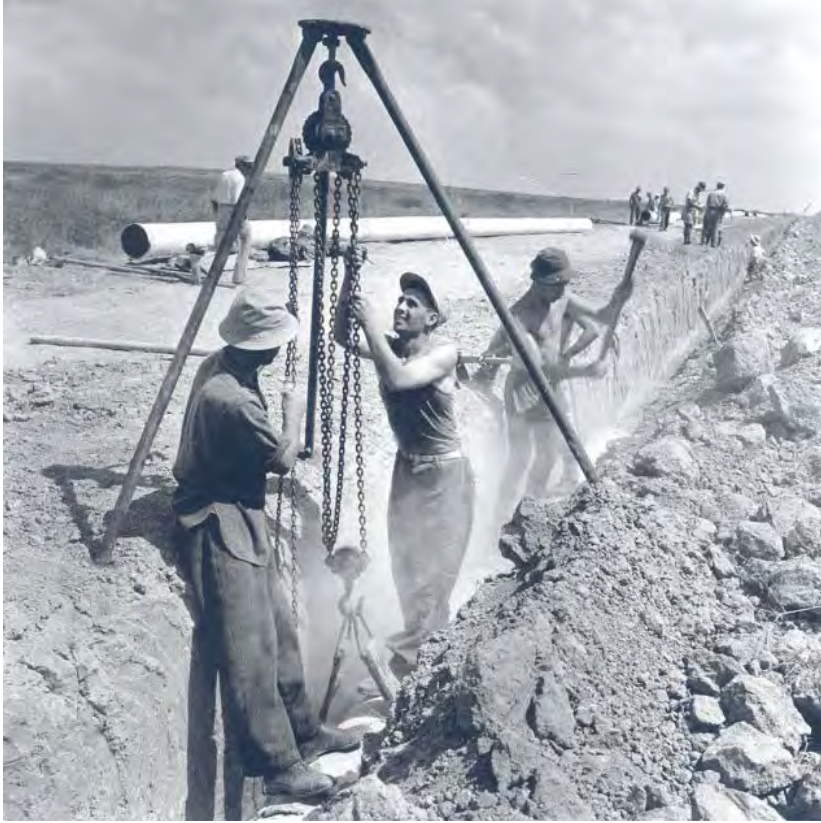
Figure 57 workers installing water pipes in the Negev, Paul Goldman 1949 Paul Goldman Press Photographer 1943-1961 Israel Museum 2004
