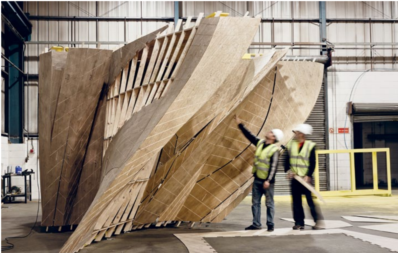
Above: Fabricators with a section of Slipstream under construction at CSI factory in Hull
