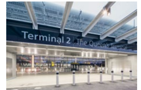
Top: Slipstream in all its glory. Above: Top-level entrance from vehicle drop-off point
