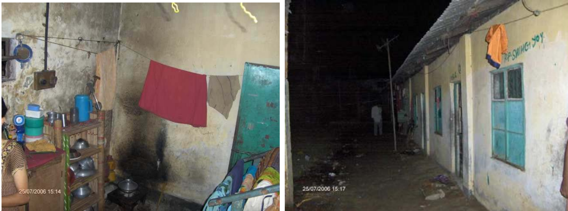
One storey mess building shared room housing
