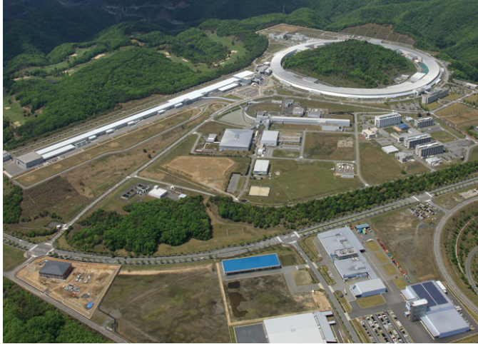
Figure 3.2: An air photo of the SPring-8 site. The figure is taken from Ref. [22].
