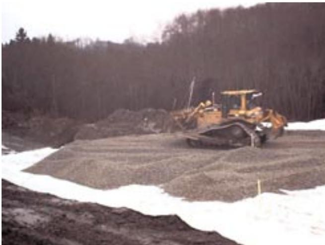
Figure 12: Distribution and compaction with dozer.
