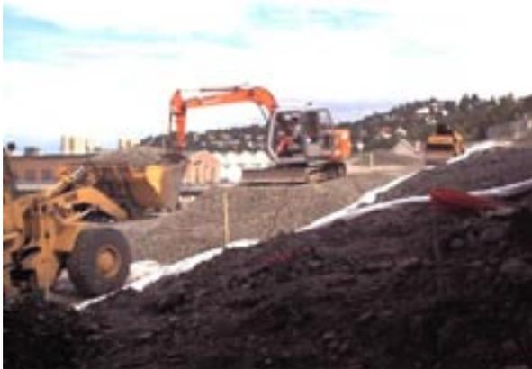
Figure 5: Distributing foamglass material using a crawler mounted excavator (Hitachi EX60, 8 tonnes). For internal transport on site a shovel dozer (CAT 923E) was used.
