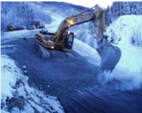
Figure 3: Placing of foamglass with excavator.
