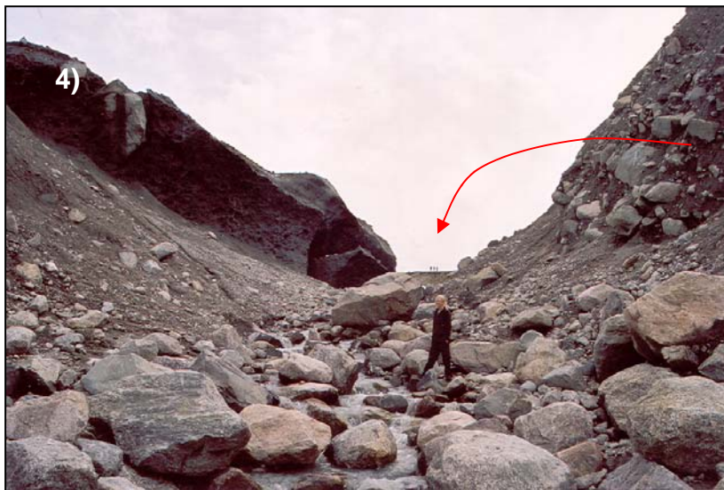
Figure 2.9 The moraine failure scar seen from downstream toe. Three persons are visible at the crest on the opposite side of the lake, and one person is in the middle of the breach.
