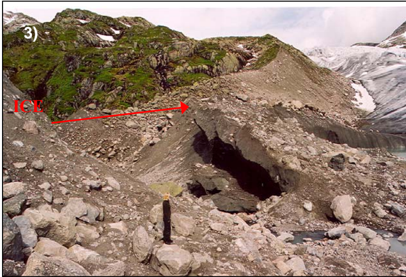
Figure 2.8 Failure seen from upstream side of dam. The ice structure in the middle of the picture may be ice transported from the glacier and covered by sediments, or an inner part of the moraine. Part of the lake is visible in the right corner.
