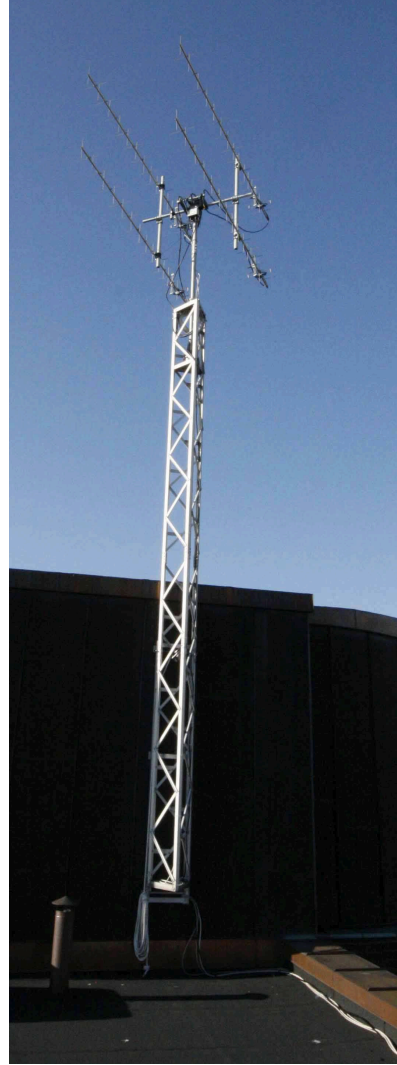
Figure 8.10: UiO ground station installation
