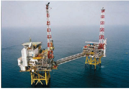
Figure 6: The Draupner wave is the first rogue wave detected by a measuring instrument. It was measured at Draupner oil platform in the North Sea off the coast of Norway on January 1, 1995 (Haver, 2003). The Draupner wave had a maximum wave height of 25.6 meters and occurred in a sea state with a significant wave height of 11.9 metres. Minor damage was inflicted on the platform during this event, confirming the validity of the reading made by a downwards–pointing laser sensor. Prior to this measurement, freak waves were known to exist only through anecdotal evidence provided by those who had encountered them at sea.
