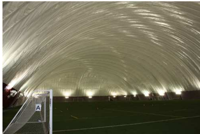
Figure 4.15: The Stinger Dome of Concordia University in Montreal
