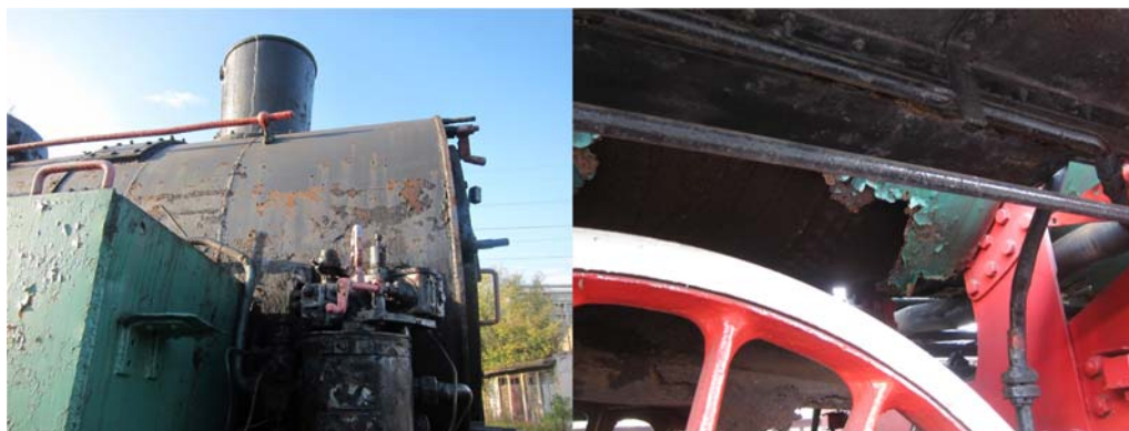
Fig. 6. Surface corrosion (left) and structural corrosion (right) on a locomotive at the Warsaw Railway Museum.
