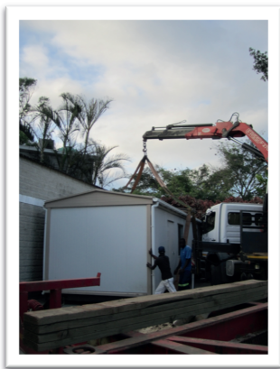
2. Building the research clinic in Ugu district.
