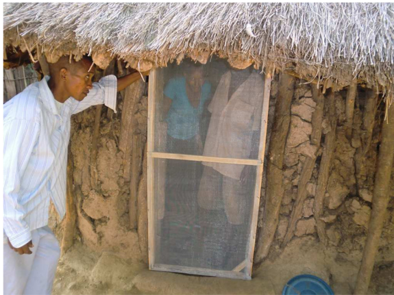
Figure 2 External view of screened door.
