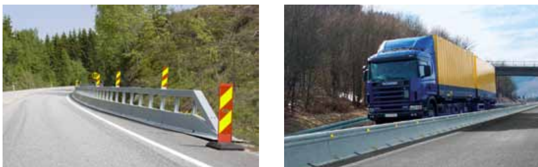
Figure 4.13 Longitudinal protection devices (examples).
