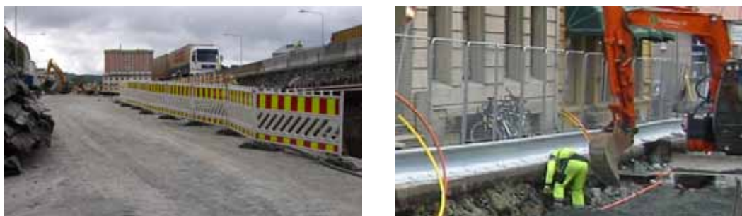
Figure 4.14 Protection devices for pedestrians and bicycle traffic.
