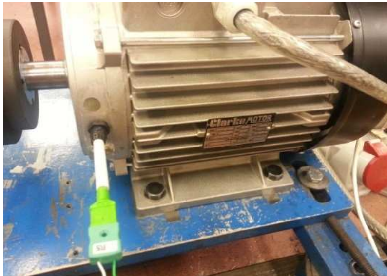
Figure 6.1- Temperature Sensor Connected to the Motor
