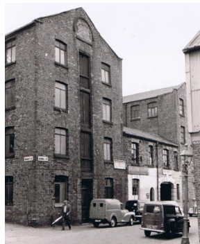
Illus. 4.1: Fairbairn & Lillie's Workshop, 20, Canal Street, Ancoats. Built 1823. 13
