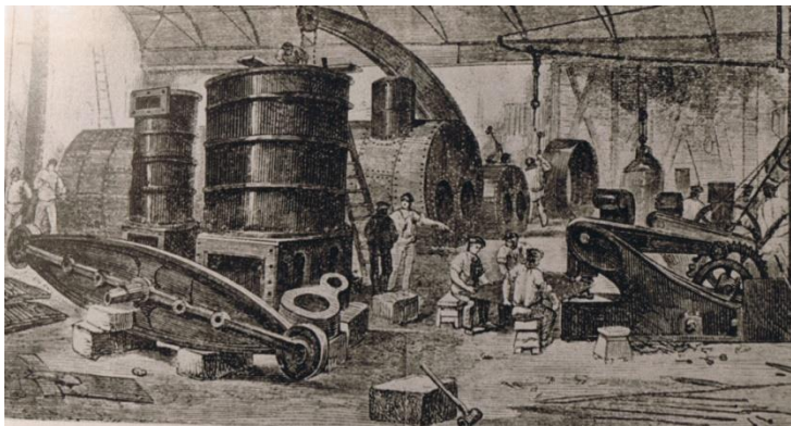
Illus. 7.13: Fairbairn crane in the company’s own boiler shop, with Lancashire boilers, c1860 195
