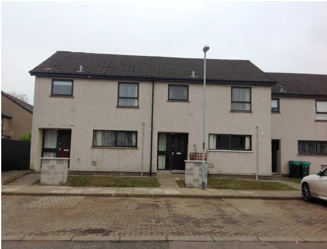
Figure 1: House 44-45 before retrofit works
