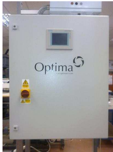
Figure 5.3 Test rig control panel.
