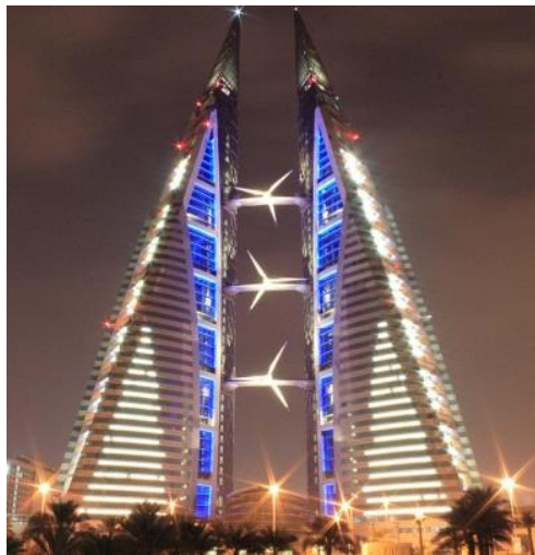
Figure 1.23: Bahrain World Trade Centre Showing Wind Turbines [1.20]
