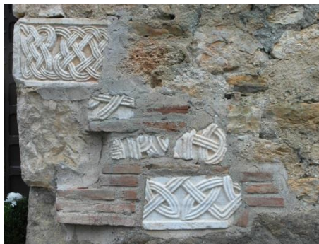
Figure 1.3: Example Ancient Stonework Used in a Modern Wall [1.1]
