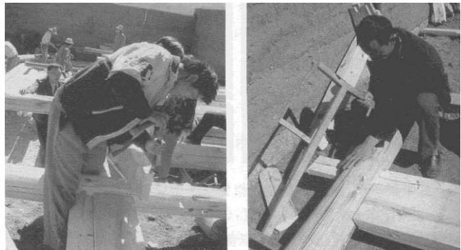
Figure 32: Assembling a timber framework on site (Bin, 2011, p.148)
