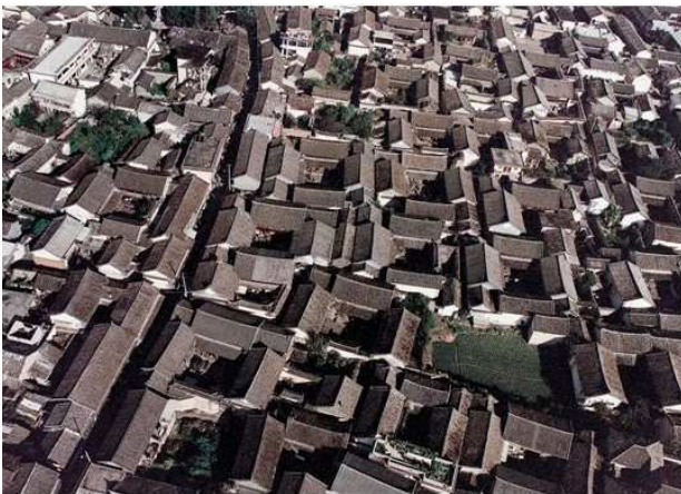
Figure 21: Aerial view of Xizhou
