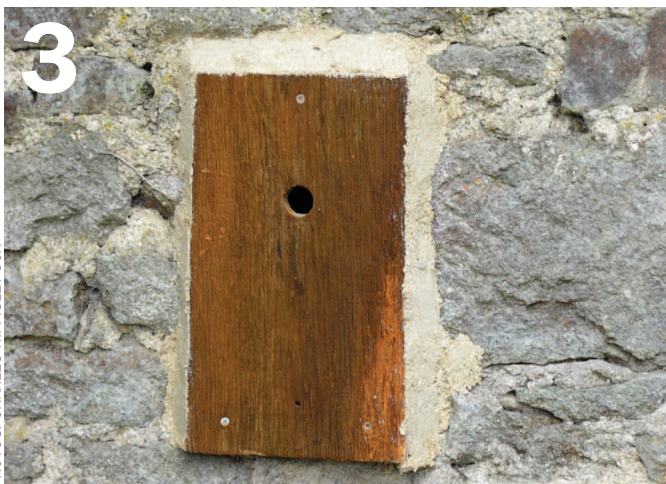
1 Use mortar to make the wall cavity the right size and shape. 2 A piece of old floorboard cut to size makes a good – and free – cover for the nestbox. A 32 mm diameter drill bit was used to make the hole. You can use different sizes to attract various bird species. The British Trust for Ornithology advises the following hole sizes: 25 mm or larger for Blue, Coal and Marsh Tits; 28 mm or larger for Great Tit and Tree Sparrow; and 32 mm for House Sparrow (see www.bto.org/about-birds/nbw/make-a-nest-box ). 3 Left-over mortar can be used to seal the sides and top, while the bottom remains open to provide ventilation. Remember that you'll need to remove the cover once the birds have left to clean out the old nest.
