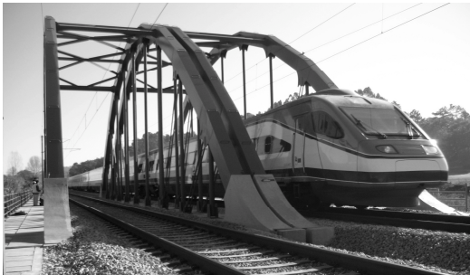
Figure 3. São Lourenço bridge and Alfa pendular train.
