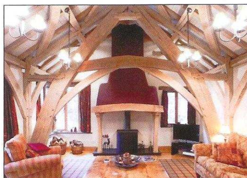
Cruck framed barn conversion in the Lake District
