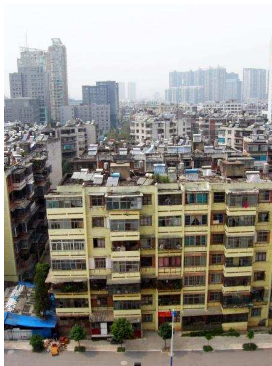
Figure 10. Solar hot water systems on roofs of residential apartments.
