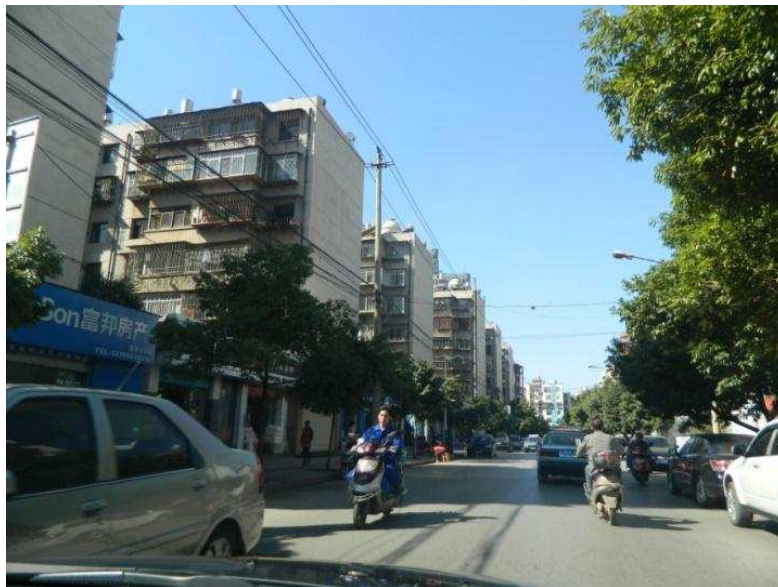
Figure 2. Typical narrow-depth residential housing.
