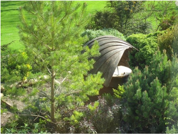
Fig 2: Cowl above inlet to earth tube
