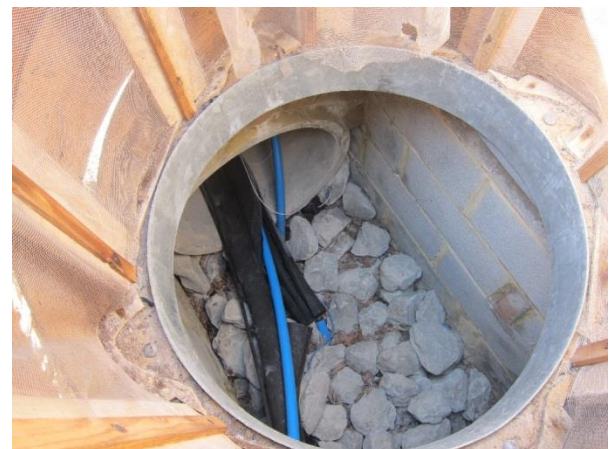
Fig 4: Junction of manhole and earth tube
