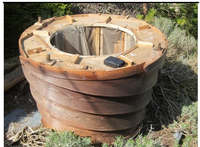
Fig 3: The air inlet terminal above the manhole
