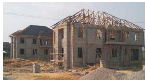
Fig 2: Building construction in Nigeria
