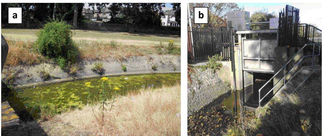
Figure 6.20 Two views of the flood management system at Mayesbrook Park: showing (a) the overflow channel between Mayesbrook and the lakes and (b) the flood sluice gate.
