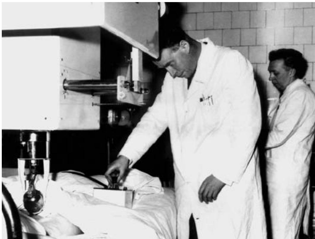
Figure 8. The first automatic scanner, designed by Tom Brown, being operated by Ian Donald and John MacVicar in the Western Infirmary, Glasgow, c. 1960.
