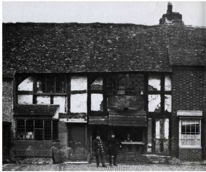
Figure 61 The house in Henley Street before restoration
