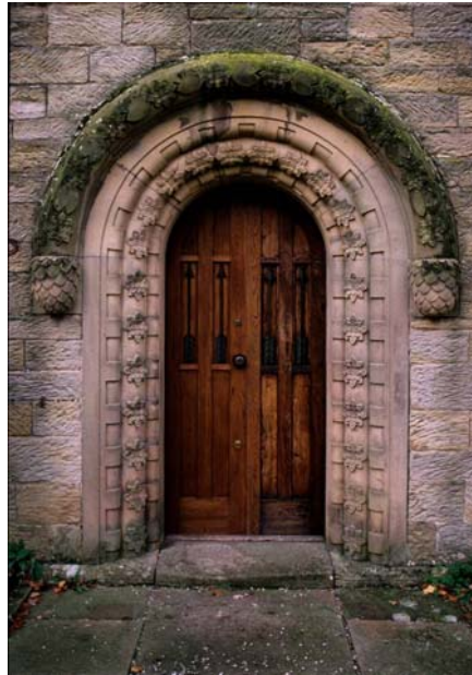
Figure 20 St Mary's Wreay, West door
