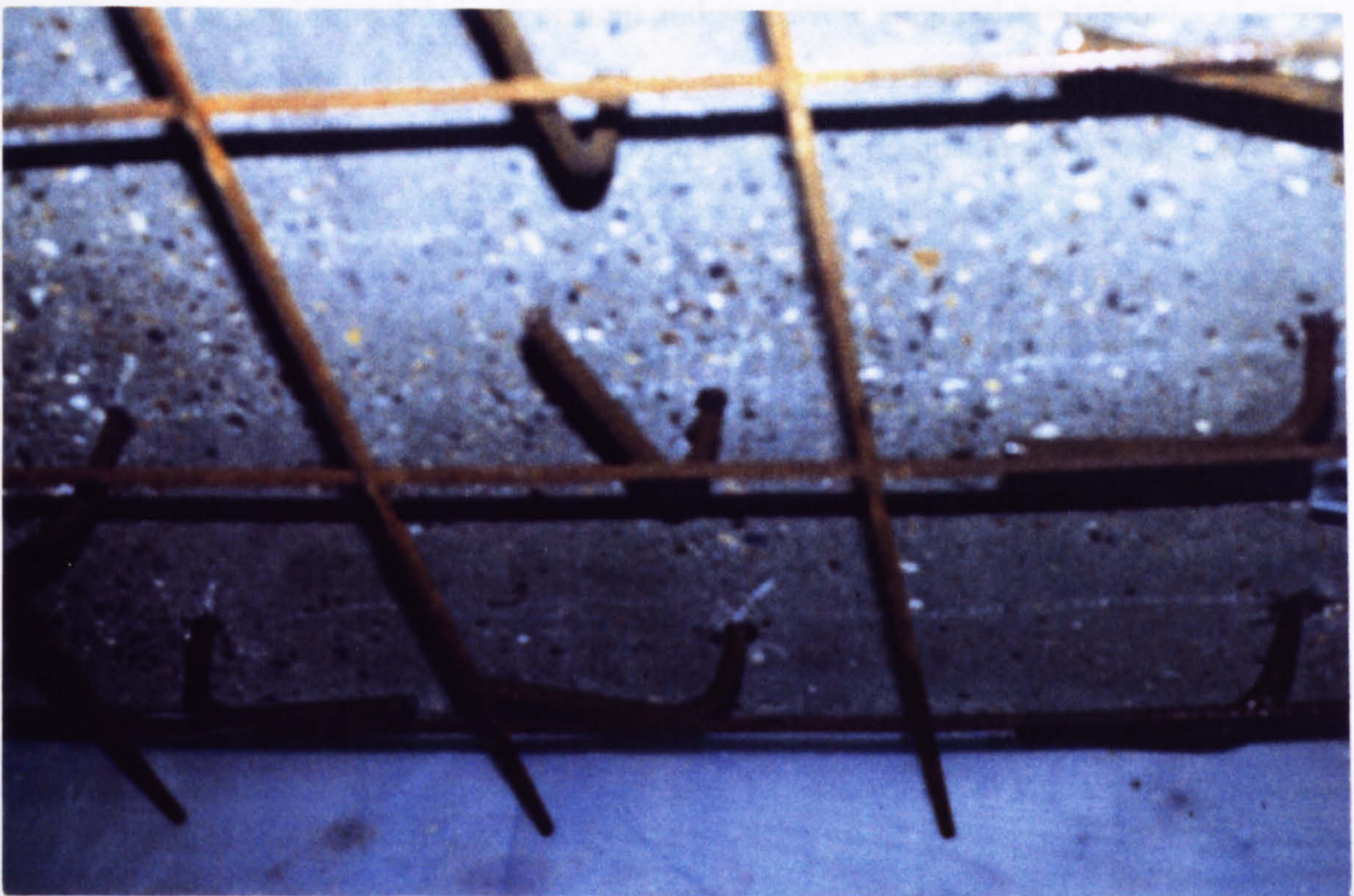
Figure 3.5a - Shear connectors fixed before the concrete spraying process.
