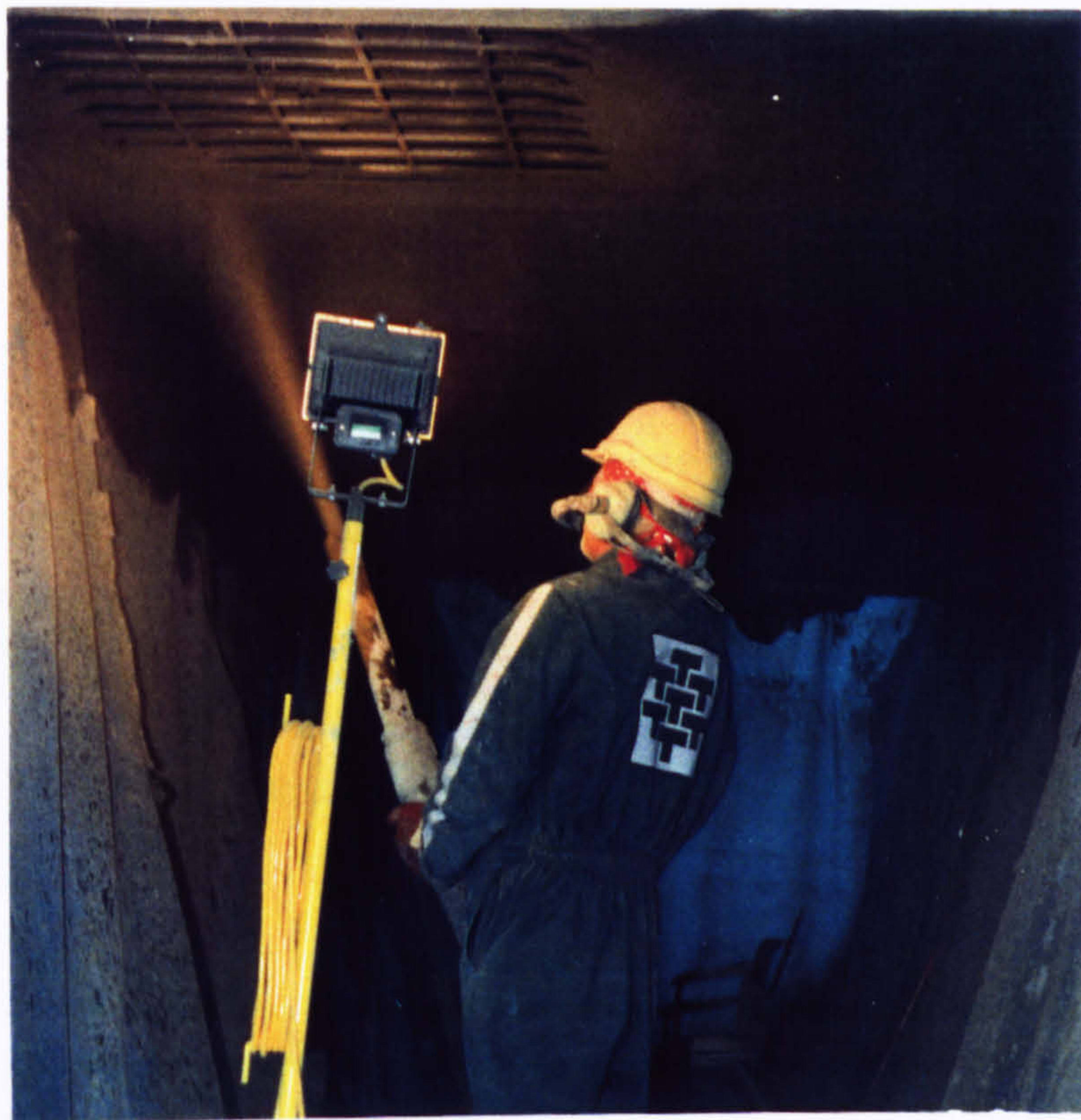
Figure 3.3b - Sprayed concrete encapsulating the mesh reinforcement.
