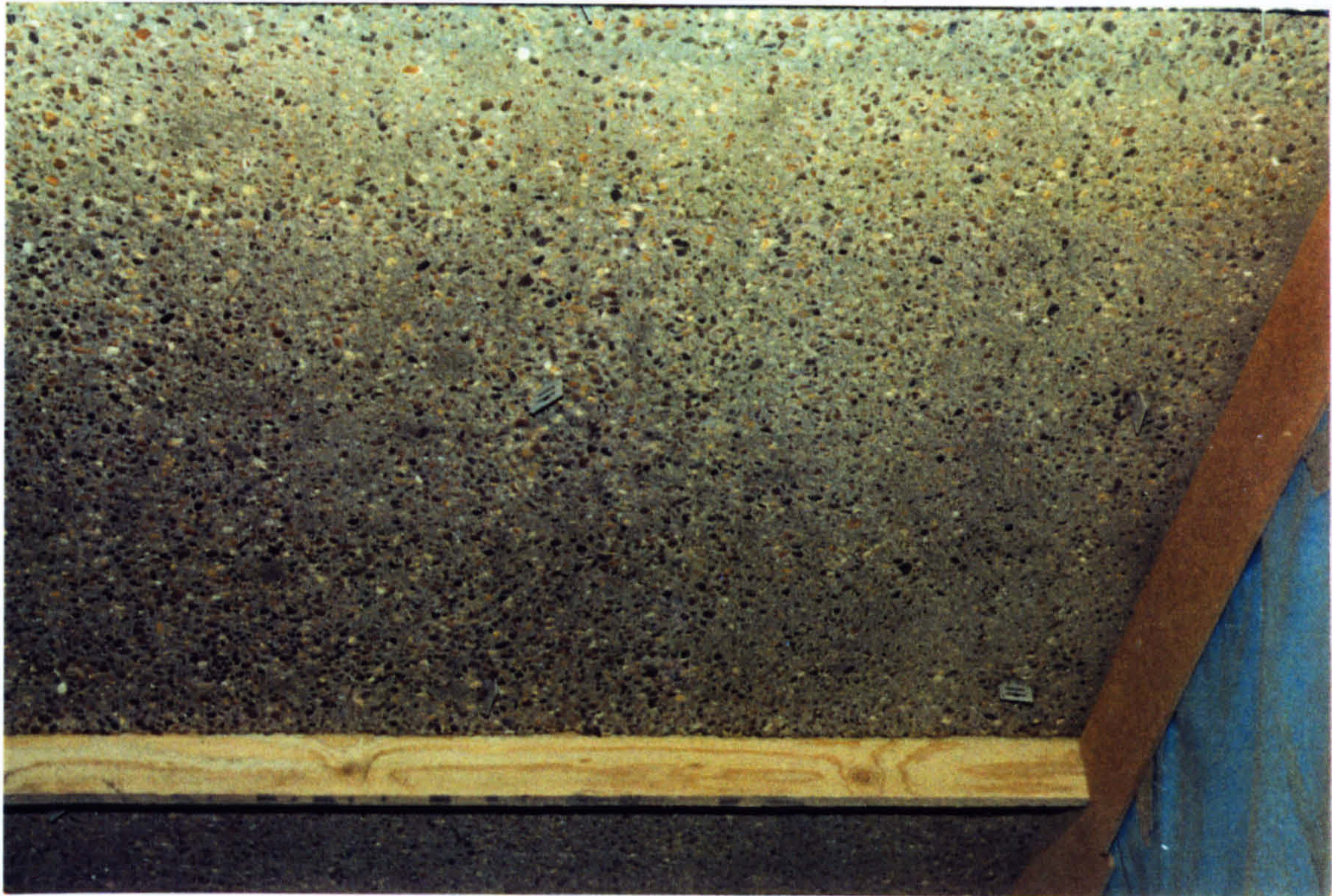
Figure 3.2c - The grit blast prepared soffit (looking from below soffit).
