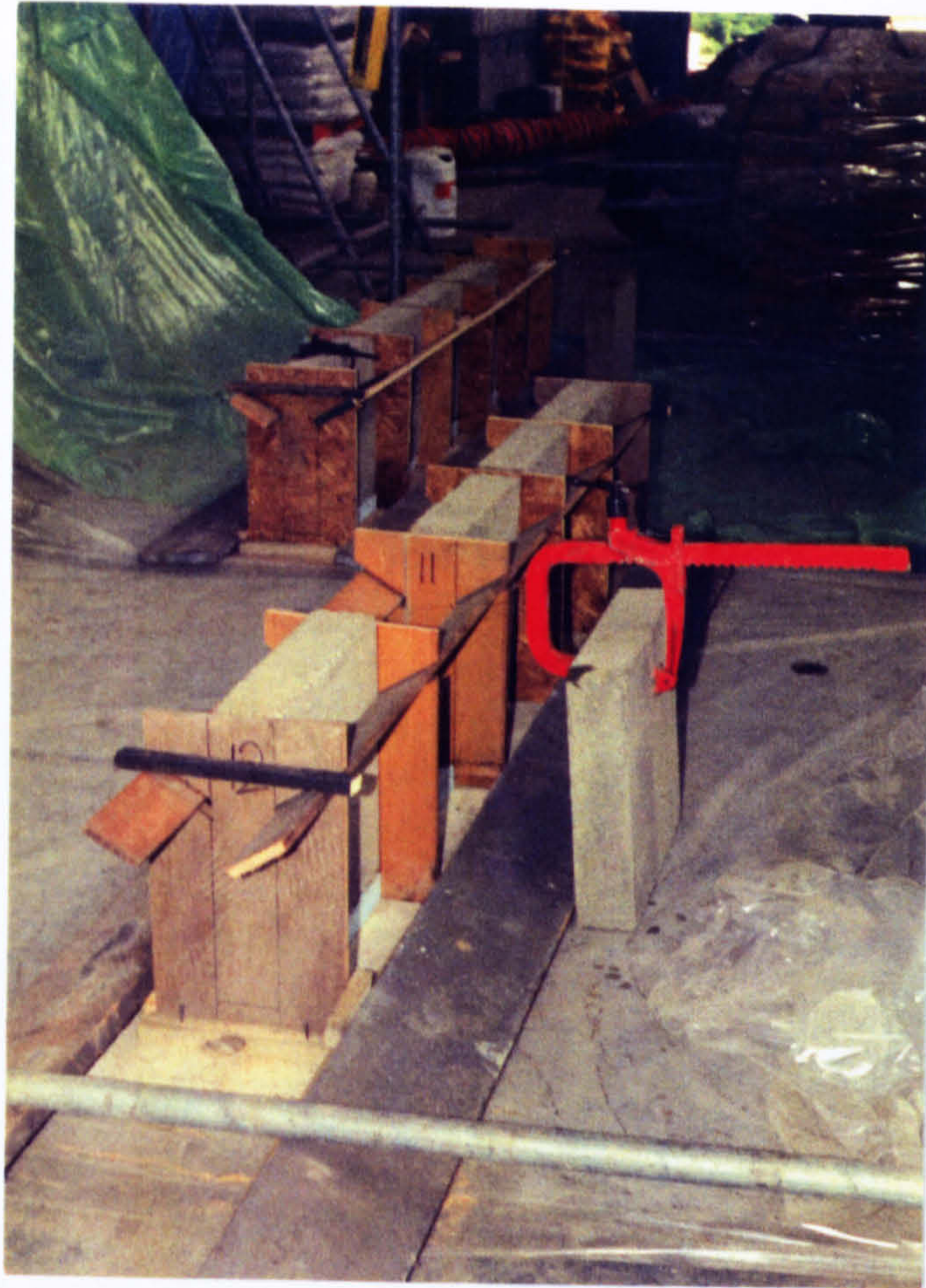
Figure 7.4a - Shuttering for the sprayed concrete parts of the double shear block.
