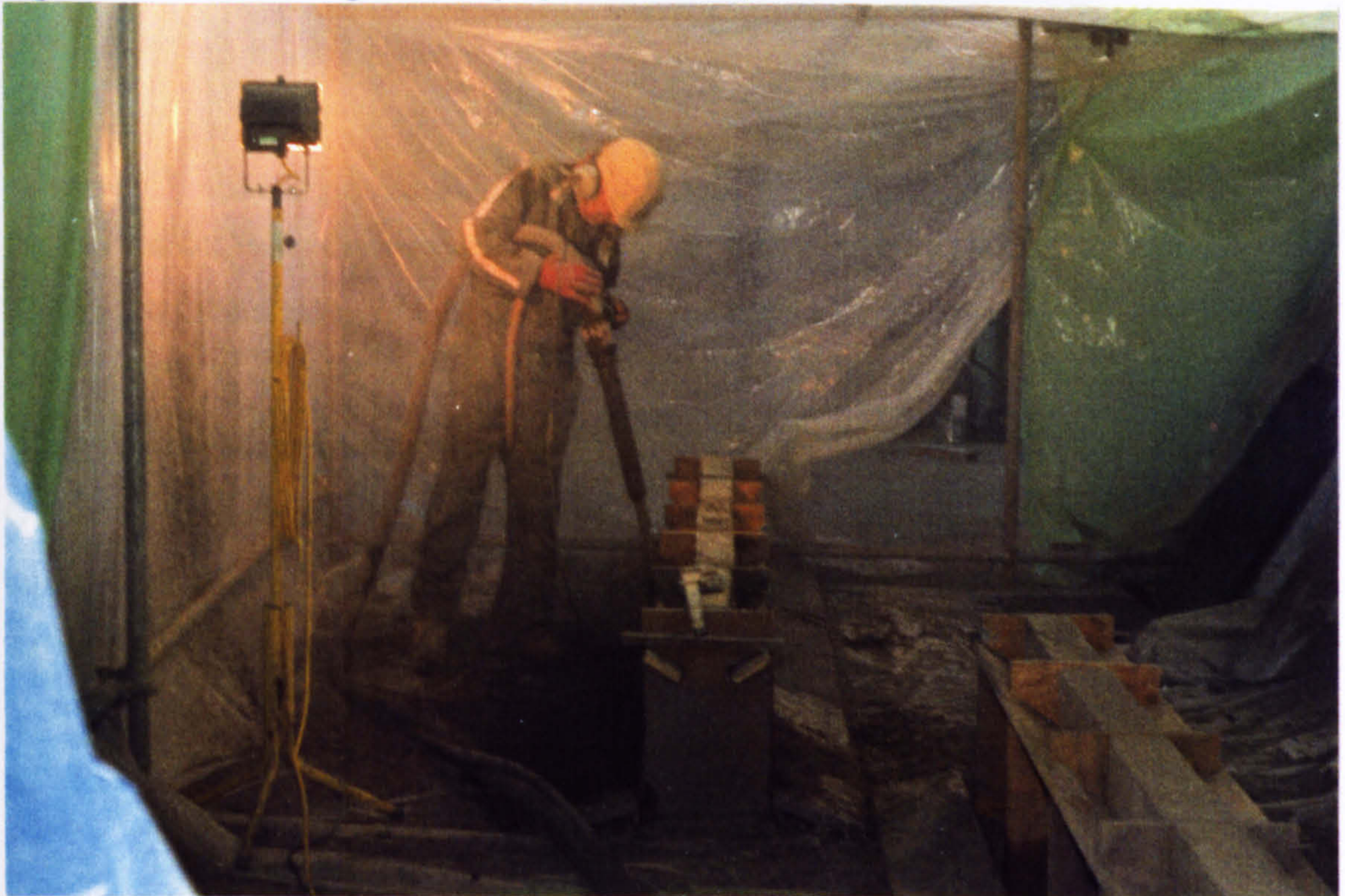
Figure 7.4b - Spraying concrete for the double block.
