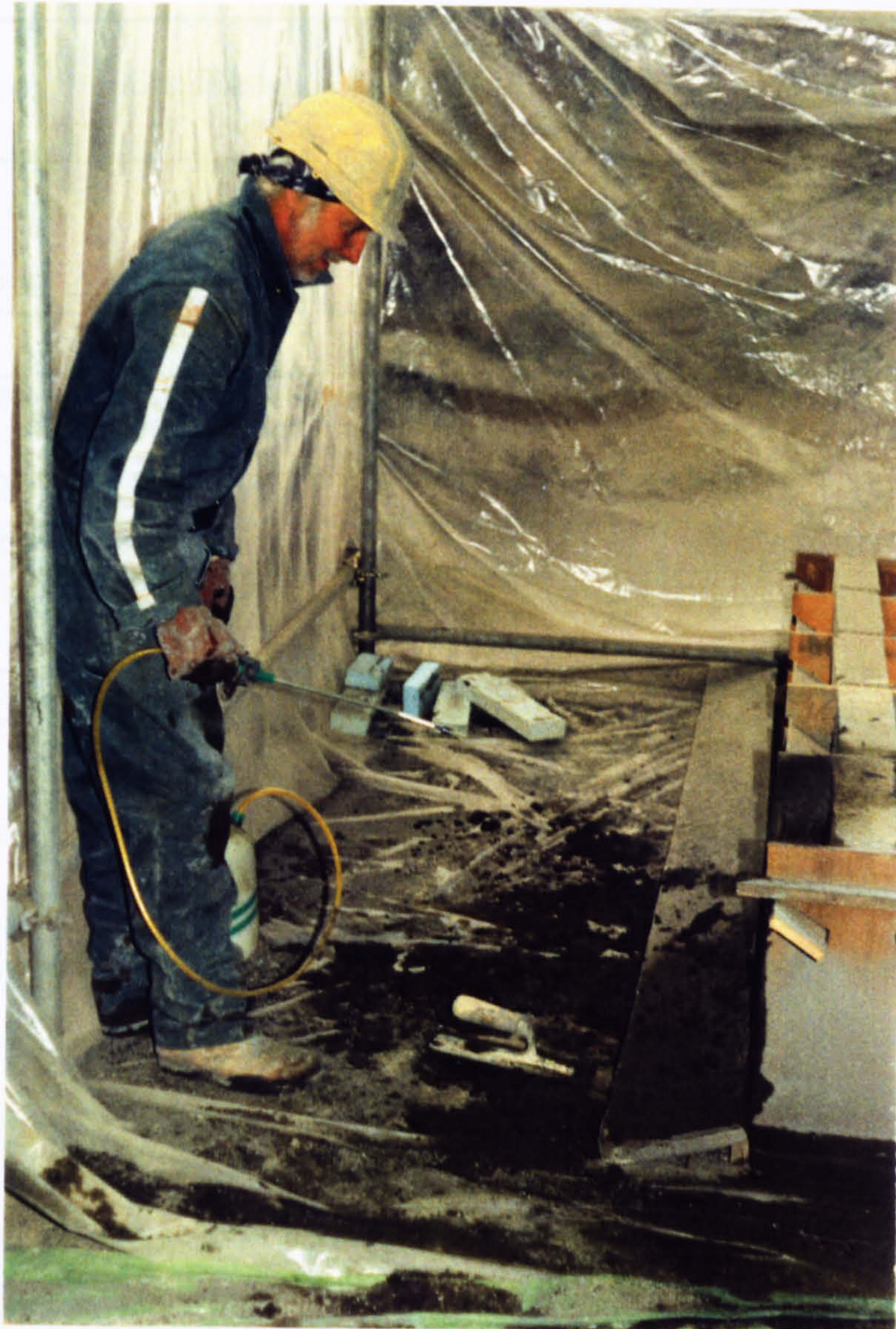
Figure 7.4c - Curing the sprayed concrete parts with a concure clear 90 membrane.
