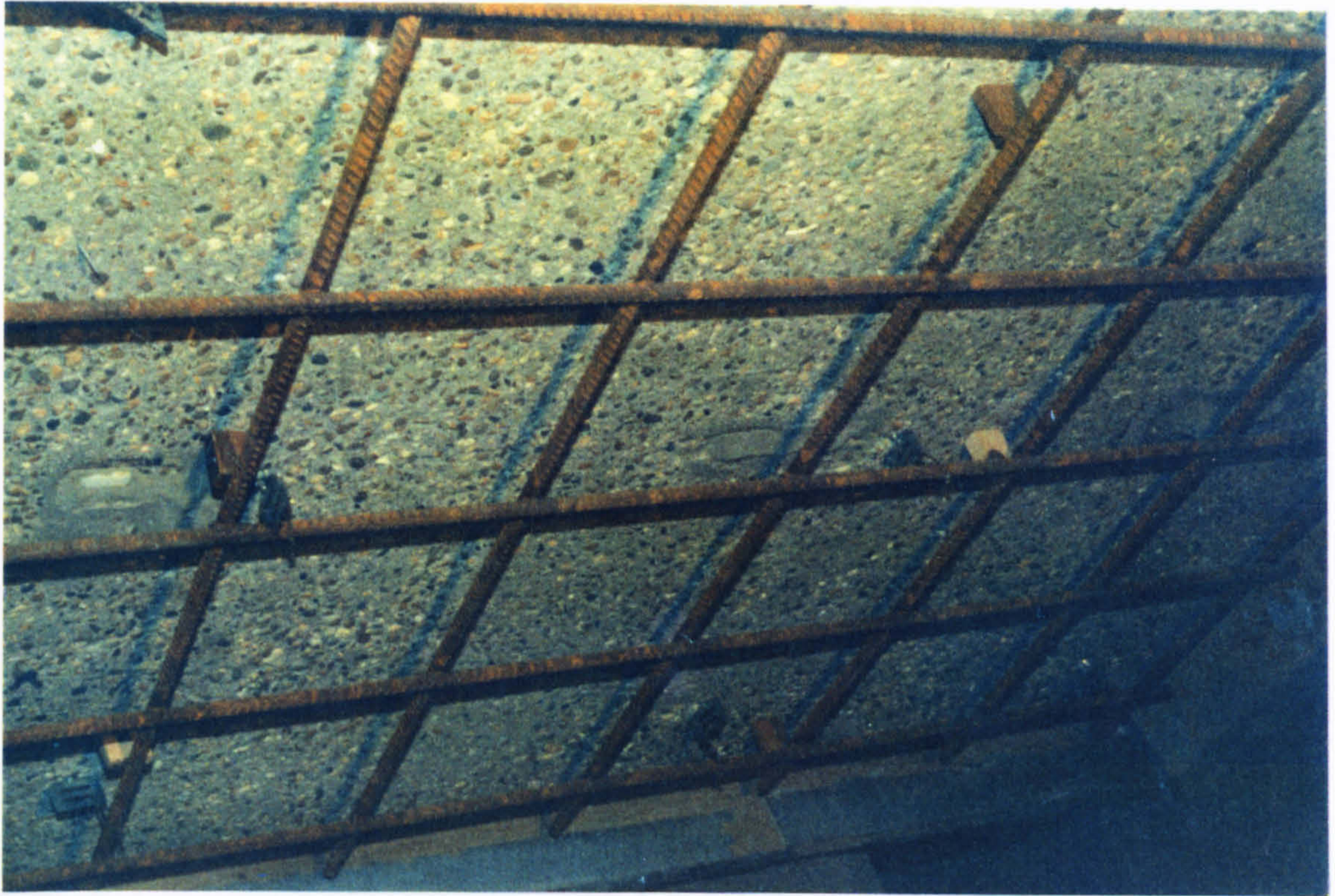
Figure 3.3a - Mesh reinforcement and spacer blocks being secured to the slab soffit.
