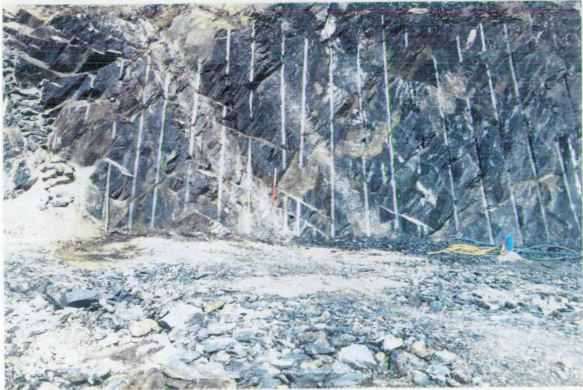
Fig. 7.7 Discontinuity structure of a cutting exposure at the A5 site.
