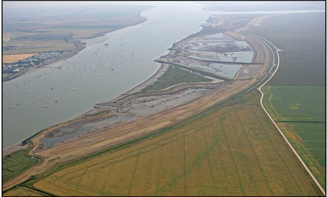
Figure 2.2 Aerial photo of Wallasea Island Managed Realignment site showing the River Crouch and the arable agricultural land. Courtesy of Colin Scott, ABPmer Limited, Southampton.
