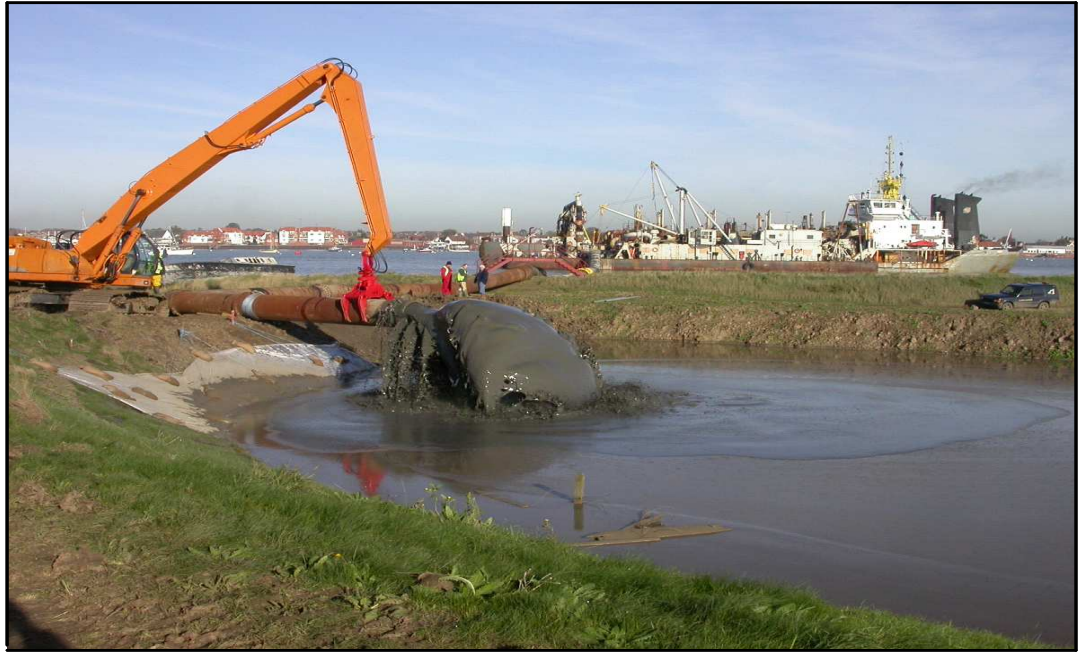
Figure 2.3 Sediment discharge into a containment bund at Wallasea Island Managed realignment site. Looking north across the River Crouch to Burnham-On-Crouch. Courtesy of Colin Scott, ABPmer Limited, Southampton.
