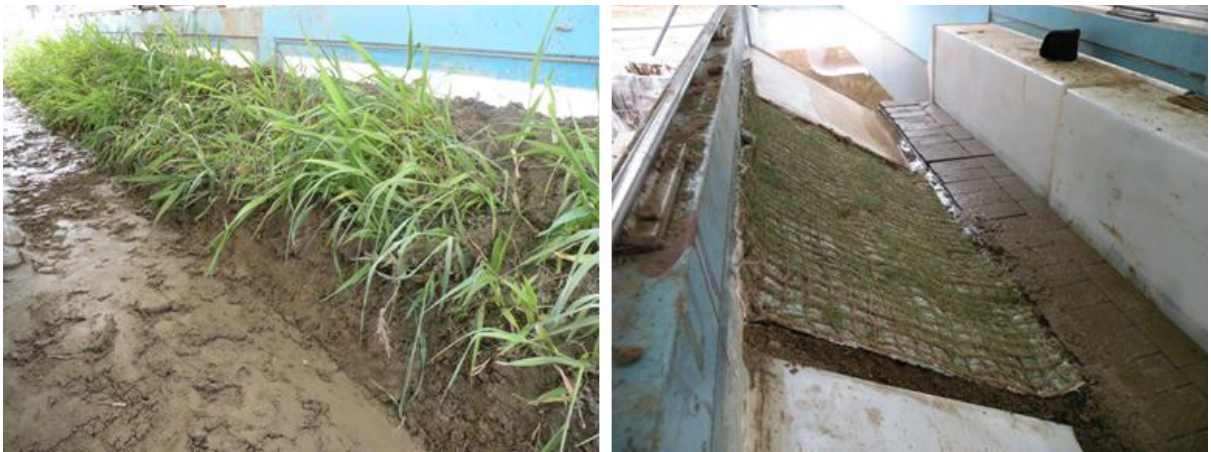
Fig. 3. Vegetation and vegetation mat installed in the channel
