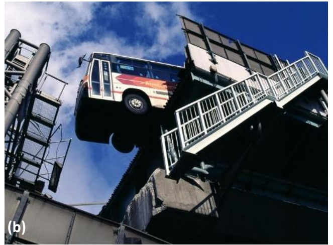
Figure 1. Direct and indirect consequences of an earthquake: (a) collapse of the Fukae section of Hanshin Expressway Route No. 3 during the 1995 Kobe earthquake; and (b) bus stopping just before a collapsed bridge span.
