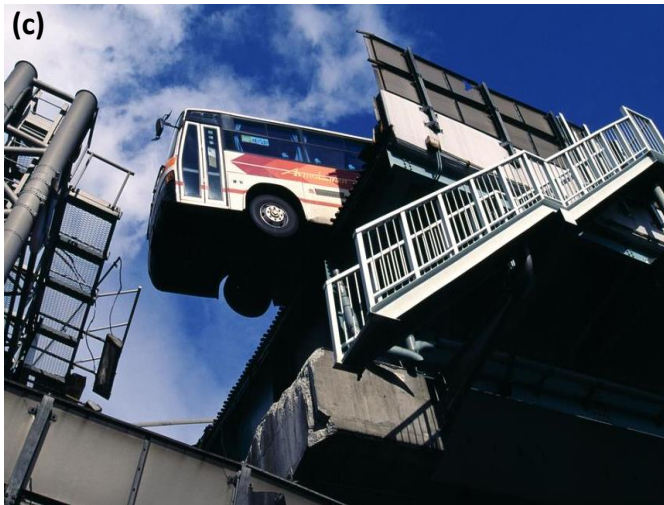
Figure 1. Structural damage of motorway bridges during: (a) the 1994 Northridge earthquake, and (b) the 1995 Kobe earthquake; (c) bus travelling on Hanshin Expressway Route No. 3 marginally stopping before a collapsed bridge span; and (d) deterioration of serviceability due to closure of road segments.
