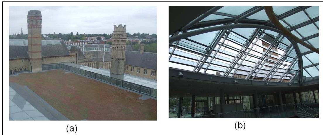
Figure 2: Example of sustainable features at Newton Arkwright Project, Sedum roof (1) and tinted glass with automatic control to improve ventilation in warm conditions (b).
