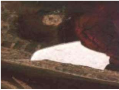
Figure 4. Detailed image of paint loss on the ceiling (shown in Figure 3) imaged from a distance of 12 m (the image corresponds to an area ~6 cm wide)
