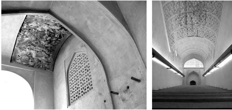
Figures 4, 5. Original stone masonry sections (left) and carved ceilings (right) stand out against the purposely rendered surrounding surfaces.
