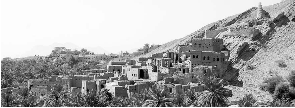
Figure 6. The eastern fortified boundary of Hārat as-Saybanī with the soaring watchtower at the top.
