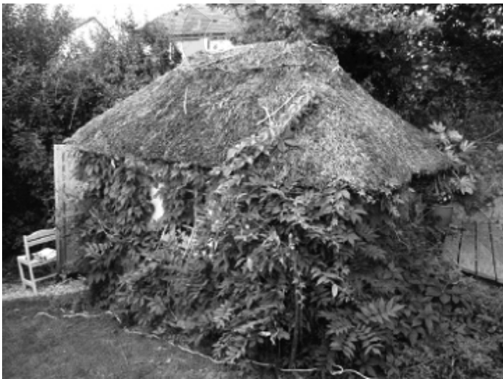
Figure 8. Building three, Summerhouse, Bovey Tracy, Devon
