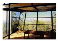
Fig. 20: Insect Meshes in Place of Conventional Walls in the Rozak House, Lake Bennett, NT, 2001
