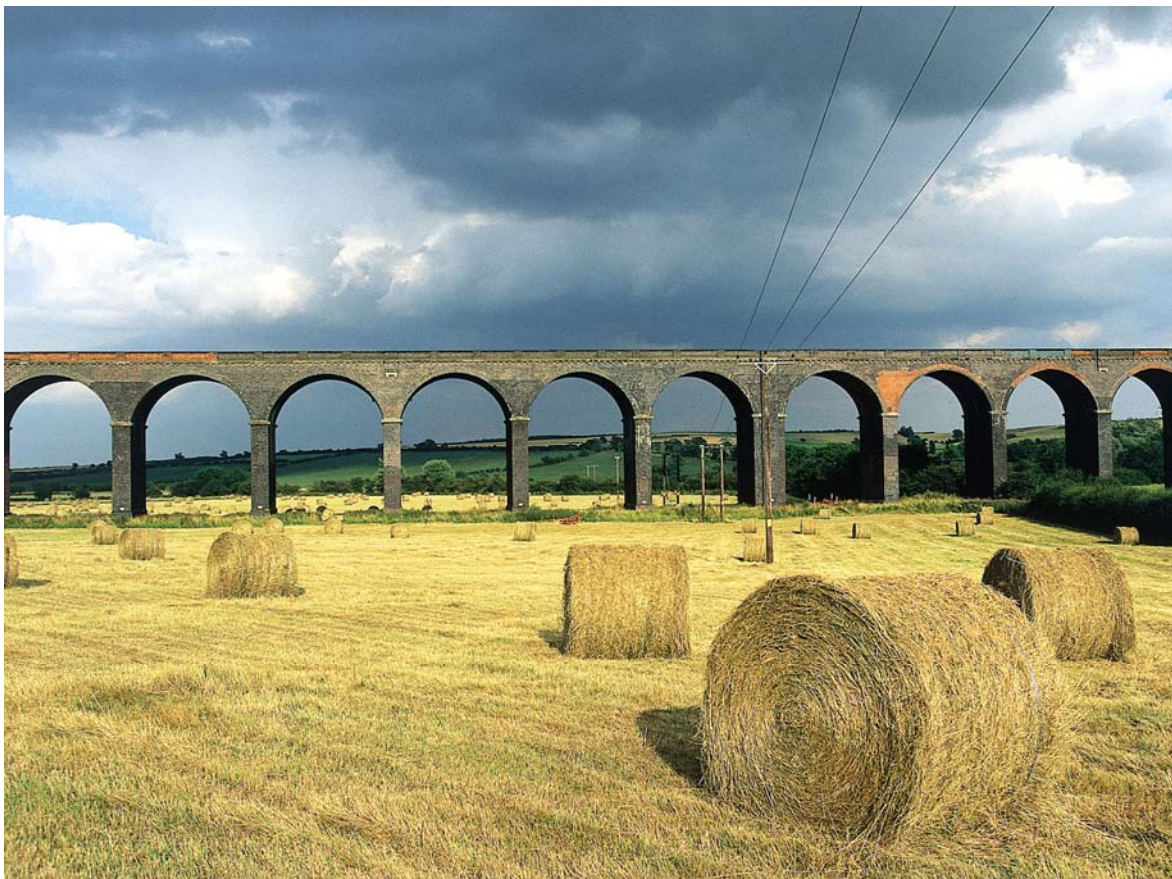
Pictured: Seaton Viaduct, Rutland.
