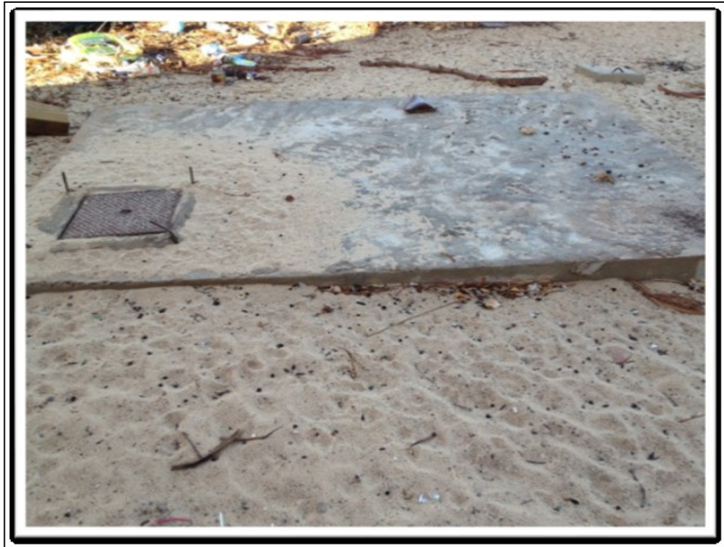
Figure 18: Septic tanks where the householders discharge wastewater in Alwaha (photo by the author 2010)
