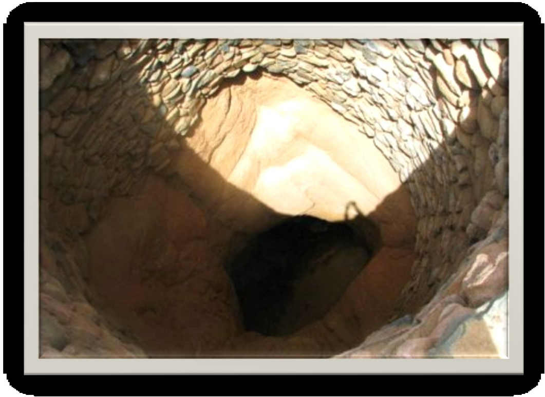
Figure 22: Unused old dug wells in Alwihat area, not used because of drying up or high salinity.
