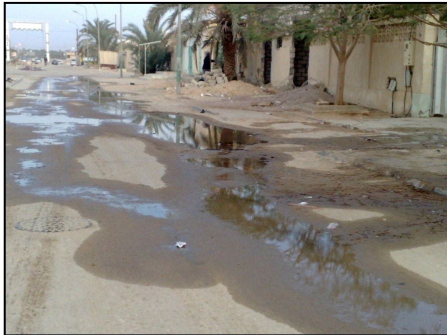
Figure 11: Evidence of urban water waste in Alwahat, 2010 (photo by the author).
