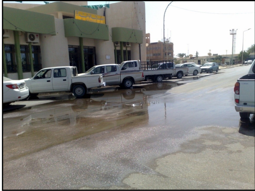
Figure 10: Evidence of urban water waste in Alwahat, 2010 (photo by the author).
