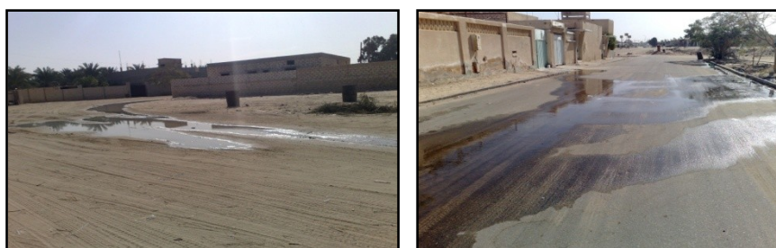
Figure 4: Evidence of urban water misuse in Alwihat (photos by the author, 2008).
