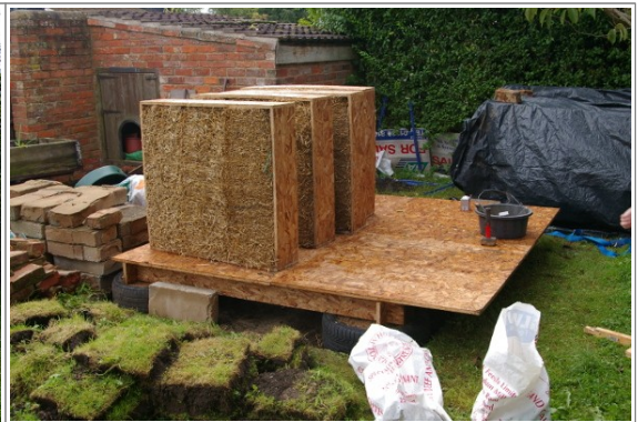
Figure V.6: Car tyre foundations, flooring, with 3 half bale loaded Blocks
