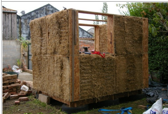
Figure V.7: Erection of Blocks (note bales are place vertically)
