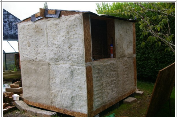
Figure V.8 Application of second layer of render
