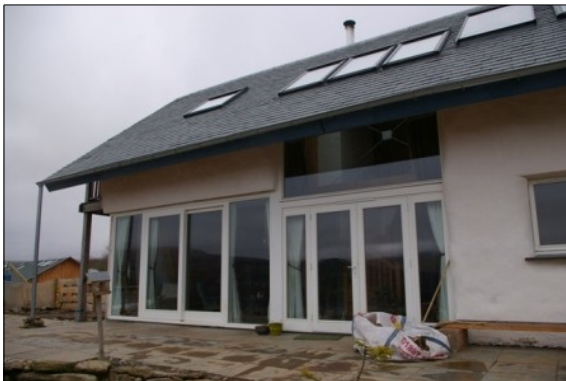
Figure IV.2: View of South-east façade
