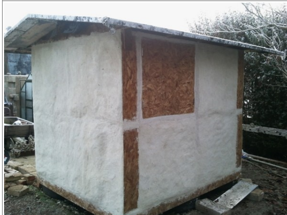
Figure V.9: Rig construction finished view from NW
