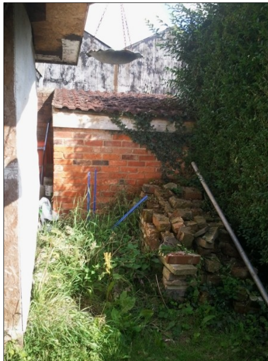
Figure VI.18: South facing elevation of Test Rig
