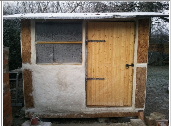
Figure V.10: Rig construction finished view from East
