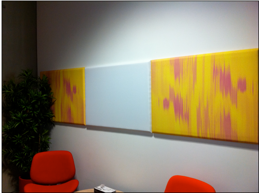
Printed acoustic panels for student counseling rooms, Newton Building, Nottingham Trent University
