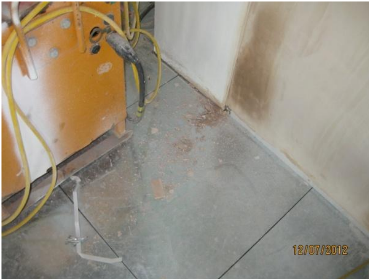
The Machine obstructing the other works – Work flow and interference
