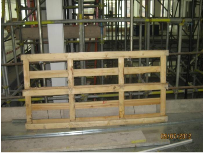
The Scaffolding delaying the other trades – Space and Connecting work
